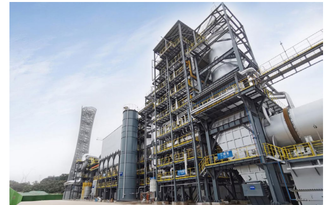
Appearance of the disposal center
